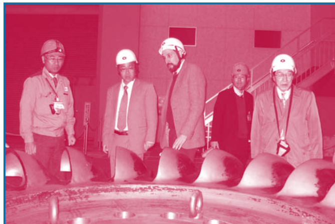
IEEE History Center Director Michael Geselowitz at Kurobe Power Plant
