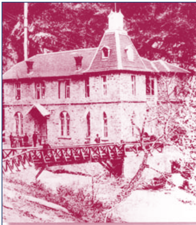
Vučje Powerplant #2 as it looked when it was built
