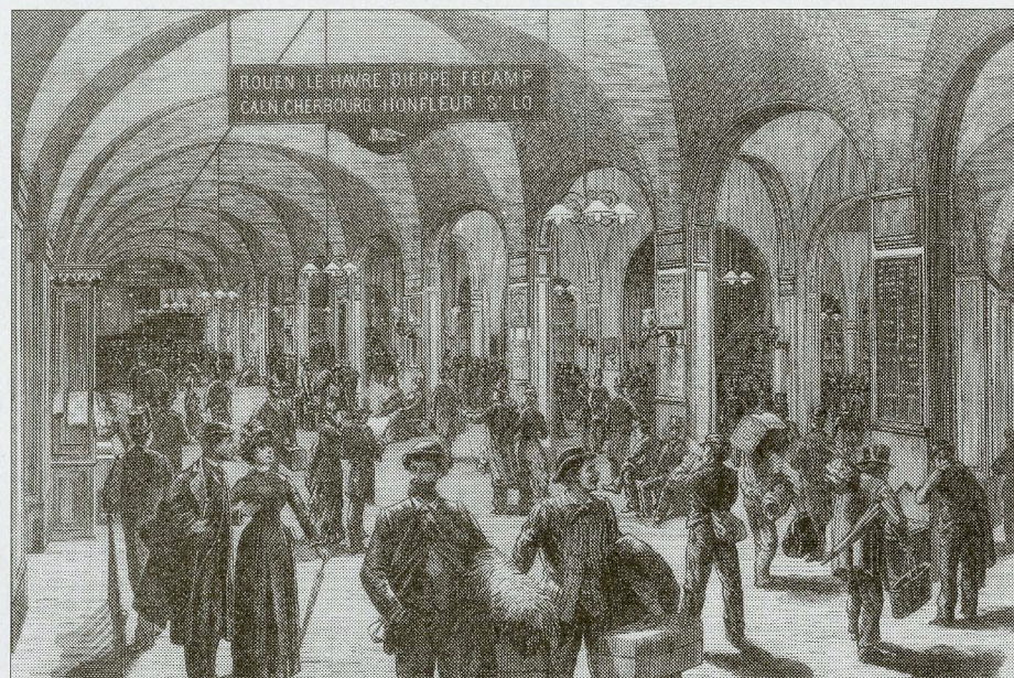
Edison lights installed in late 19th century French railway station.
