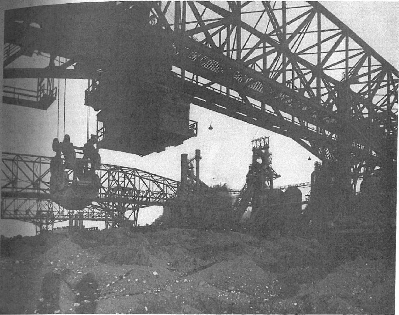
Shown in the background are two of the newest and largest blast furnaces which were just put into operation at the South Chicago works of the Carnegie-Illinois Steel Corp. These two furnaces can each produce 1500 tons of iron a day and are part of United States Steel Corp.'s $875,000,000 post war development program.
