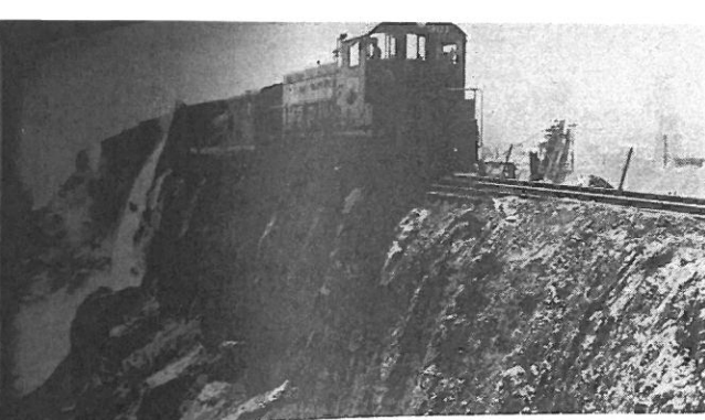
These slag pots in a southern mill are being dumped by means of compressed air instead of by steam as used to be normal practice. Since this train is run by a diesel locomotive a special car is attached to the locomotive which compresses air for operation of the slag pots.
