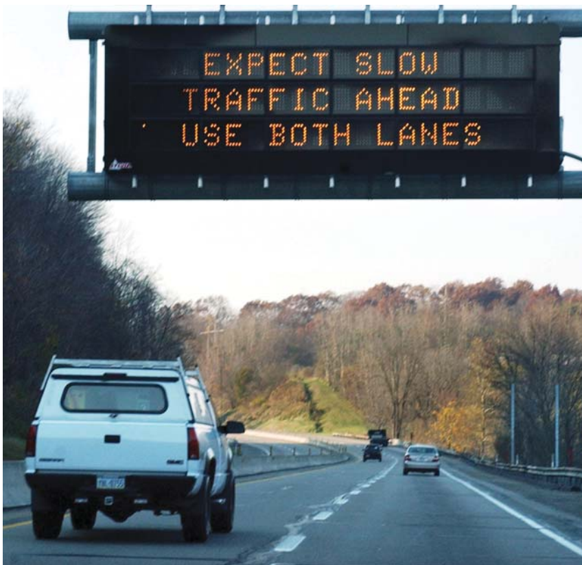
Electronic billboard on the Pennsylvania Turnpike, USA, warns drivers of traffic problems ahead. The billboard is part of a computerized information network being installed on the highway that will include cameras, weather stations, and emergency warning systems.
