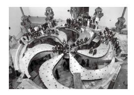
Meanwhile in the Meson Hall the 16-m diameter vacuum chamber was being assembled by Ebco. You will notice how it is festooned in coils – both for adjusting the magnetic field and for water cooling – and indeed the 54 circular trim coils were Reg's crucial tools for tuning the beam to full energy. In February 1972 the tank was lifted over the wall and
