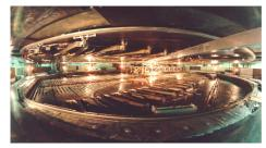
Above the cyclotron three layers of concrete beams were installed for shielding, and on top of them the electrostatic injection line from the ion sources. Within the cyclotron vault the extracted beam lines had been installed, and outside it the proton lines were complete, but the meson hall still looked very bare.
