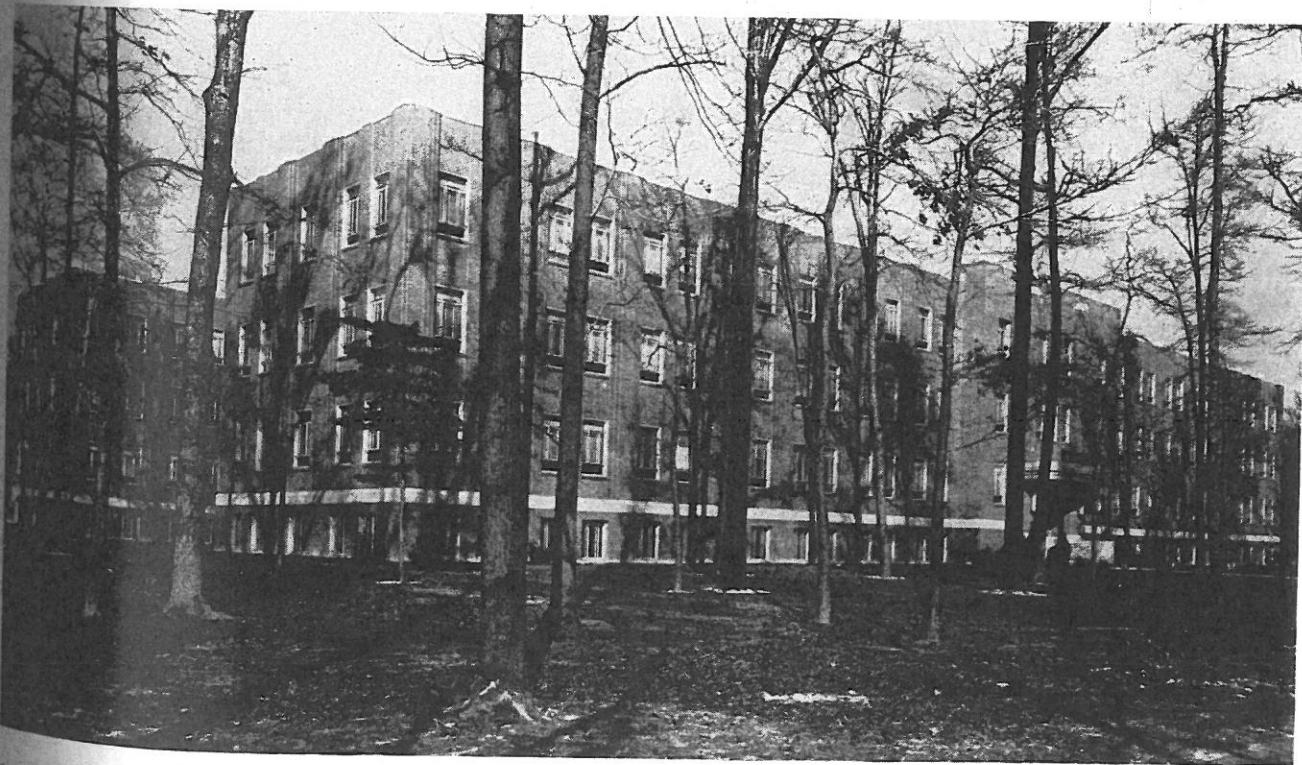
The general office at Sparrows Point, air-conditioned and modern in every respect, was completed in 1941.
