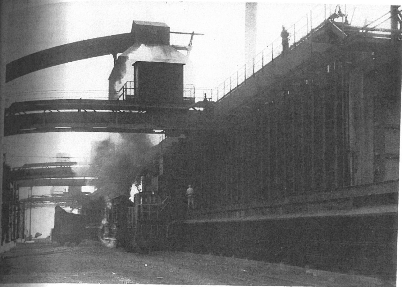
Two new batteries of coke ovens have brought the plant's capacity up to 2,520,000 net tons of coke per year.
