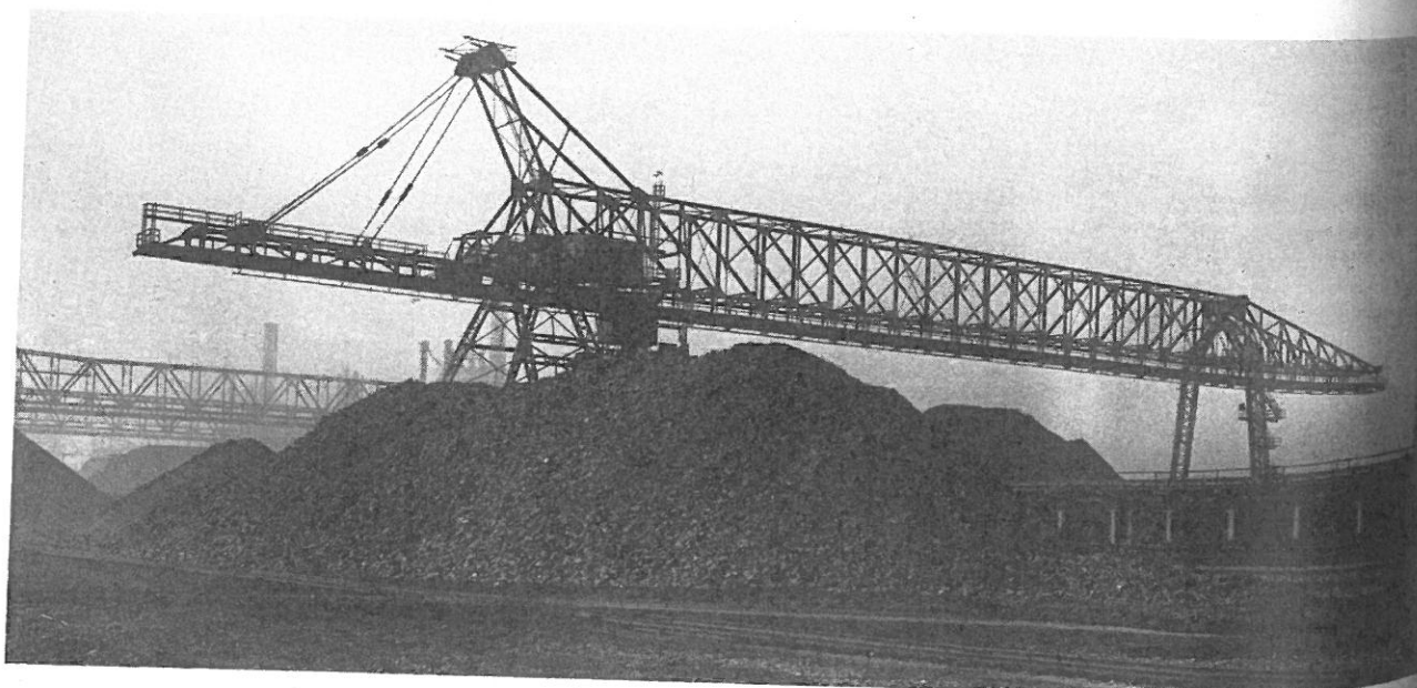
The ore storage yard, accommodating approximately 1,000,000 tons of ore, is 2500 ft long, and lies adjacent to the river
