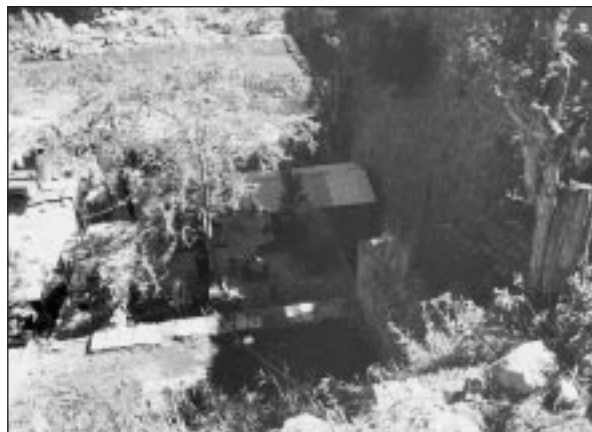
The Batopilas Stored Hydro Generating Facility seen from the wall of the aqueduct, Batopilas, Mexico.
