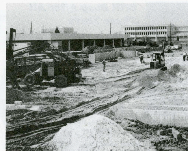
Construction of original Service Center expansion, 1979.
