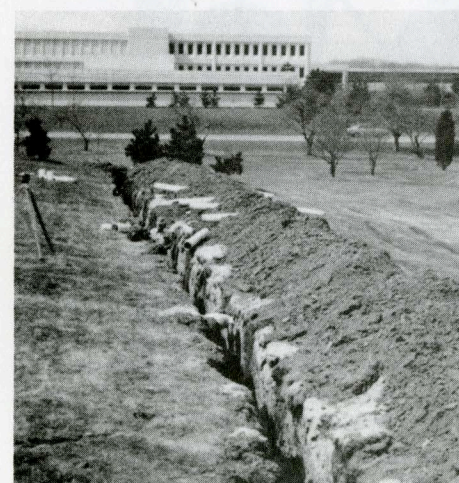
Ground Breaking of 1979 warehouse expansion.
