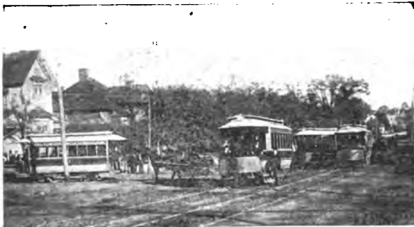
THE ATHENS, GA., ELECTRIC RAILWAY.
