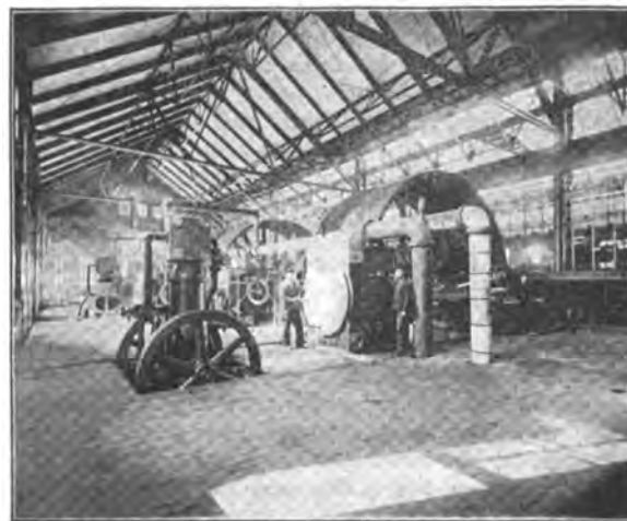
FIG. 14.—VIEW IN THE ENGINE ROOM.
