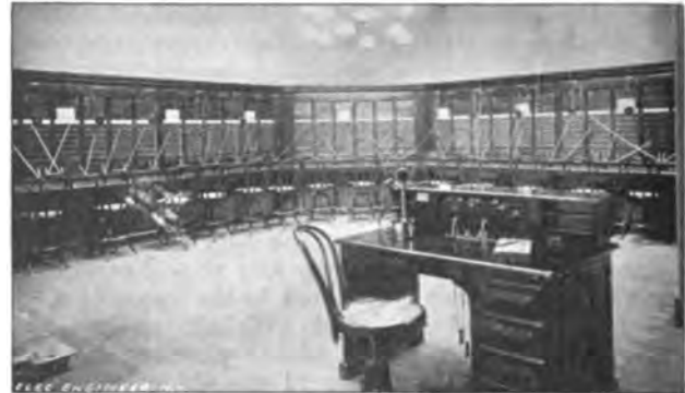
FIG. 3.—MULTIPLE BOARD AND MONITOR'S DESK, BOTH WITH CONNECTIONS UP.
