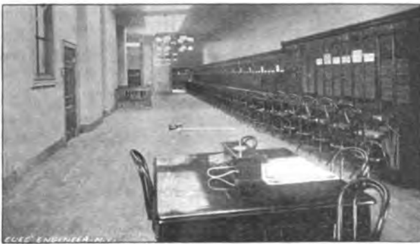
FIG. 2.—MULTIPLE SWITCH BOARD AND CHIEF OPERATOR'S DESK.
