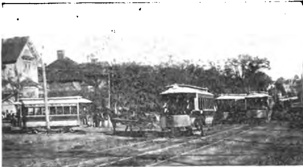
THE ATHENS, GA., ELECTRIC RAILWAY.
