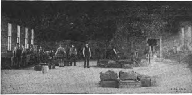
FIG. 1.—MOULDING ROOM, EUREKA TEMPERED COPPER CO.'S FACTORY, NORTH EAST, PA.
