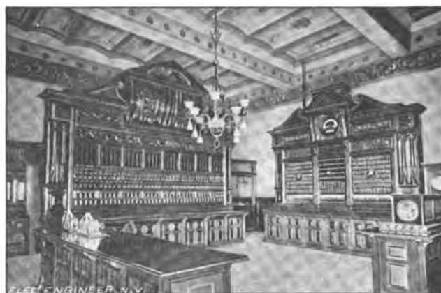
CENTRAL OFFICE OF THE PITTSBURGH FIRE ALARM SERVICE.
