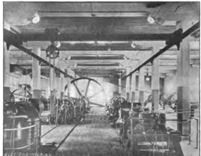
FIG. 1.—GENERATORS, PITTSFIELD, MASS., ELECTRIC LIGHT STATION.
